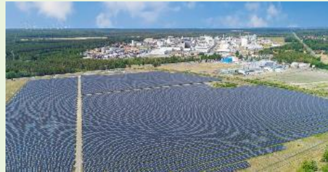
On-site solar park Schwarzheide, Germany
