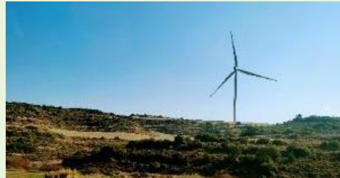
25 years onshore wind power from Spain
